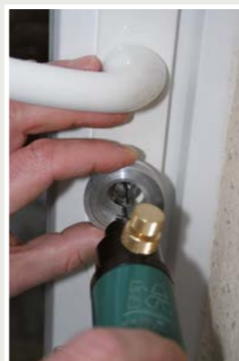
Use of the dynamometric tension tool
